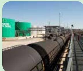
*Recycled animal fats and used oils are brought to the Diamond Green Diesel facility by truck and rail, where they are processed into renewable diesel and can be distributed with petroleum diesel via the pipeline infrastructure.*
